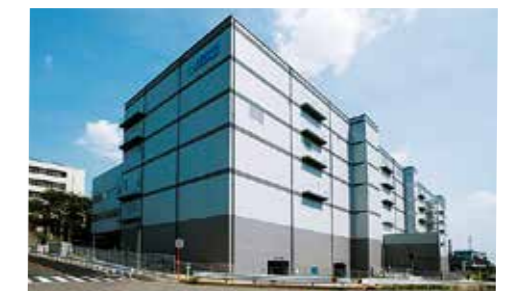
Plant for Toyota PCB Waste Treatment Facility, Japan Environmental Storage & Safety Corporation (JESCO)
